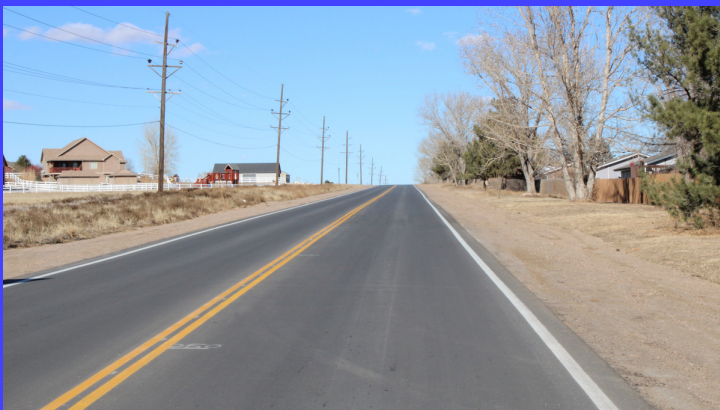
47th Avenue asphalt reconstruction
