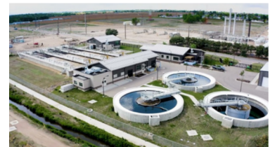
The City's Wastewater Treatment Plant will be expanded in the future.
