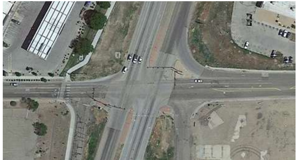
Figure 2.38: US-85 and 31st Street
