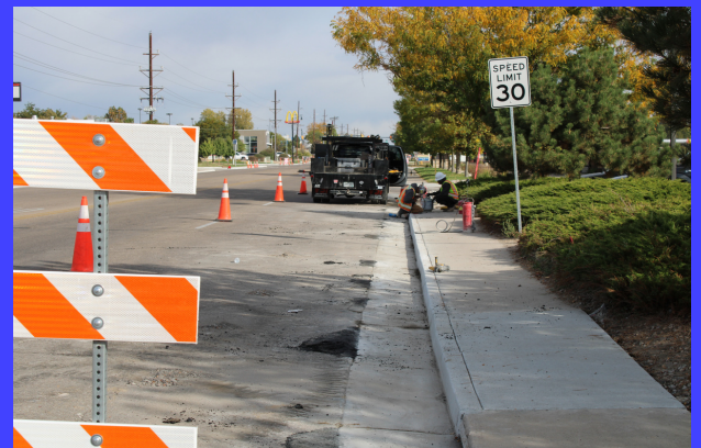
Sidewalk repairs on 23rd Avenue
