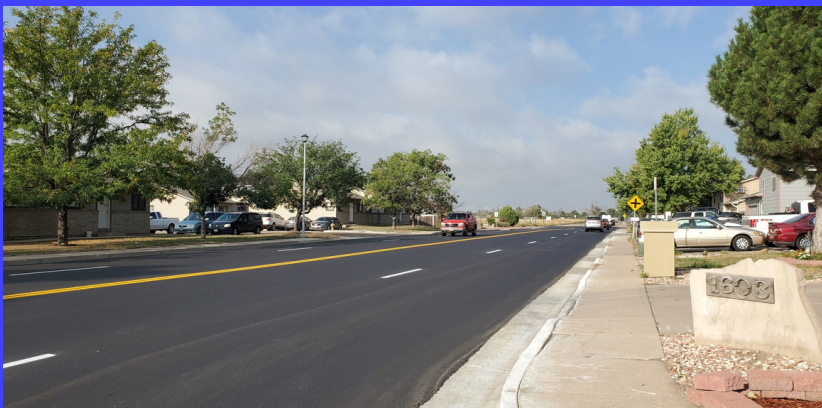
42nd Street asphalt improvements
